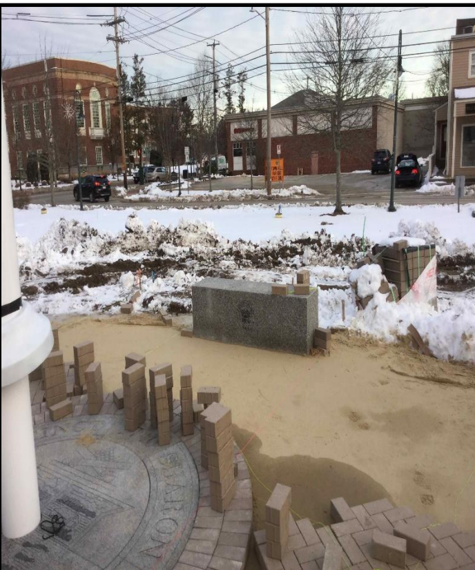
Sand and Paver Install
