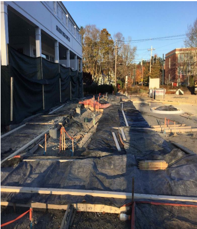
Concrete Sidewalk Protection
