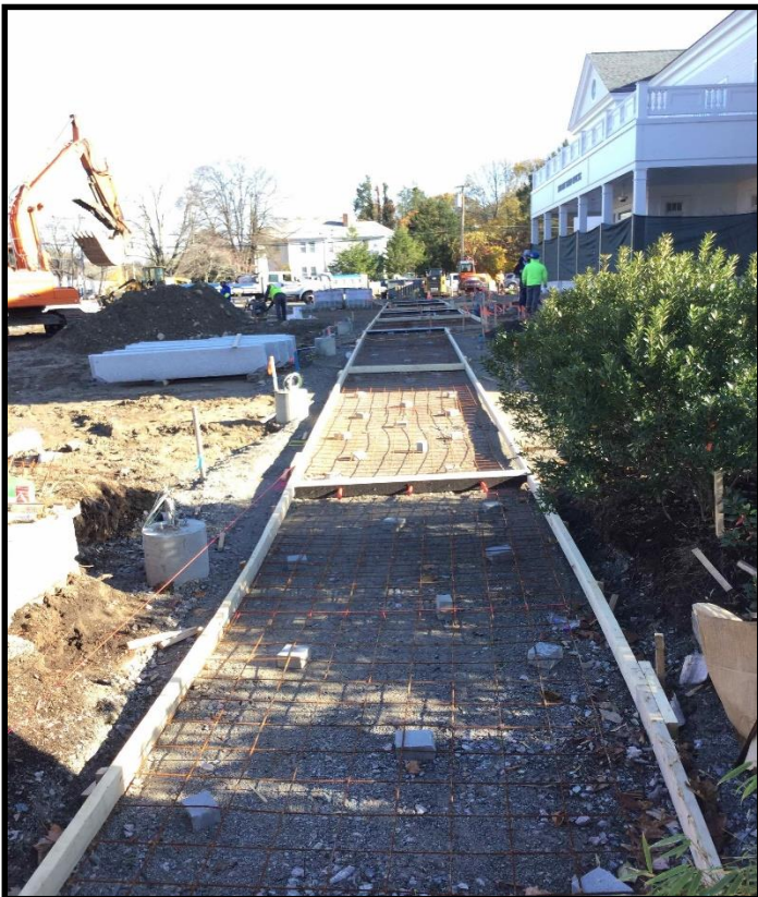
Sidewalk Reinforcement
