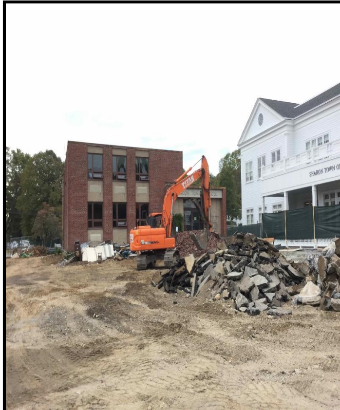
Asphalt Removal
