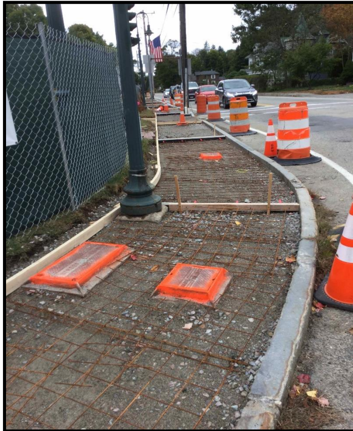
Main St. Sidewalk Reinforcement
