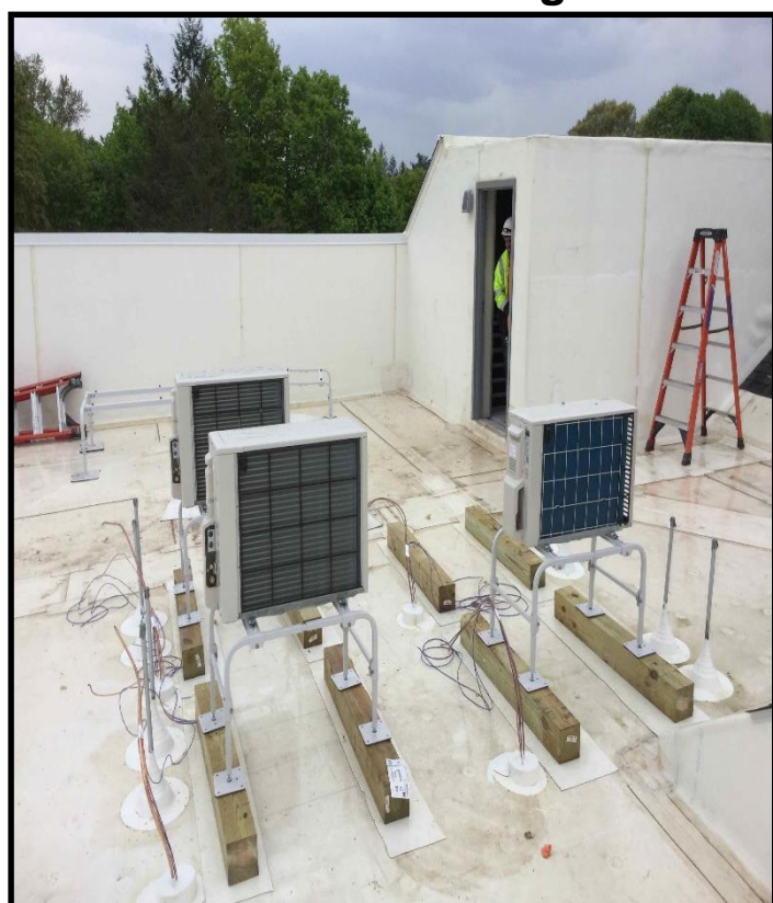
Roof Top Condensers
