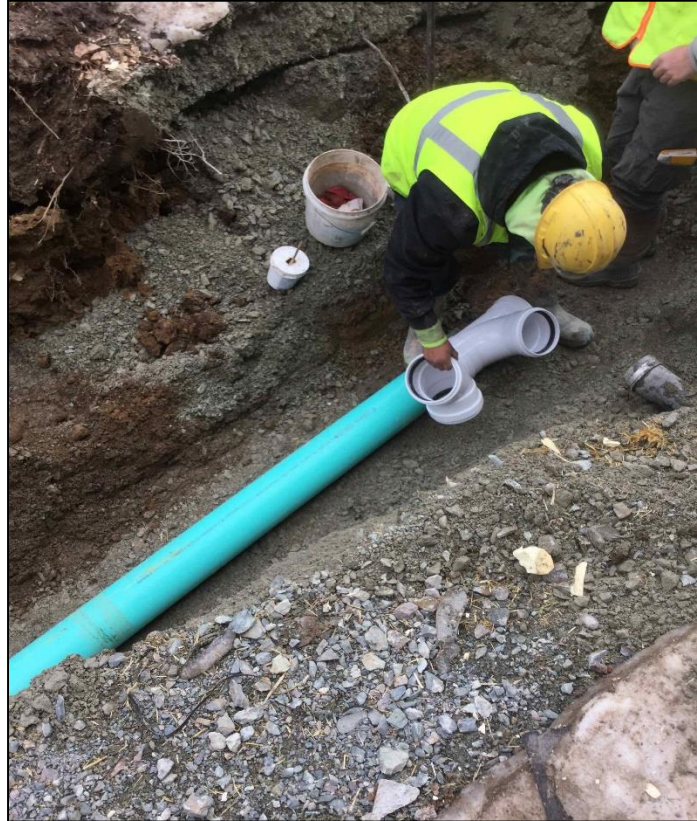
Storm Drainage Install
