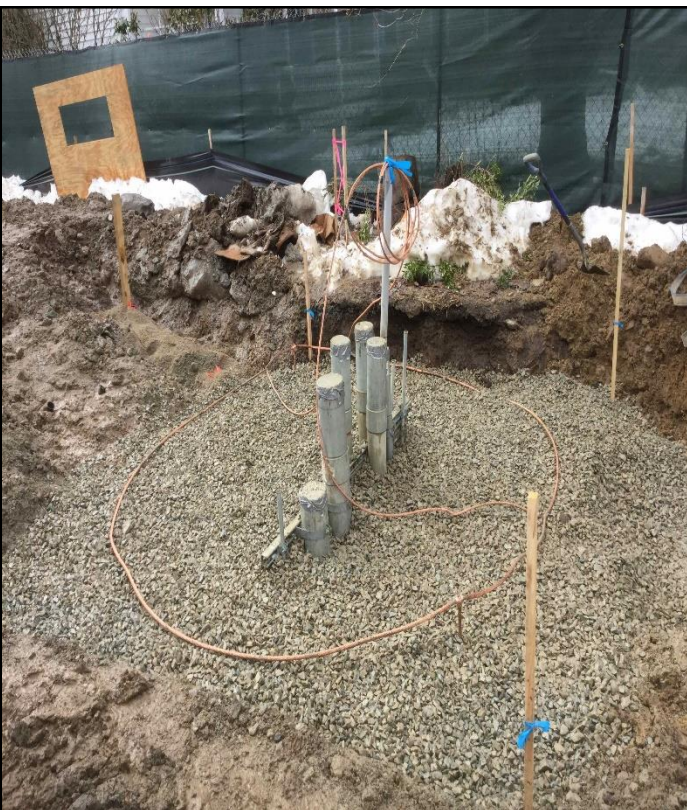
Transformer Grounding
