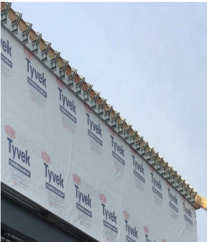
Gutter Framing
