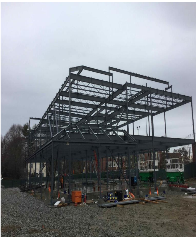
Joist Installation
