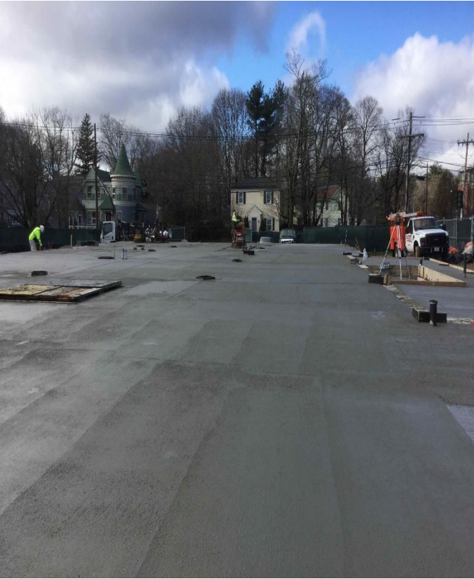
Slab Placement
