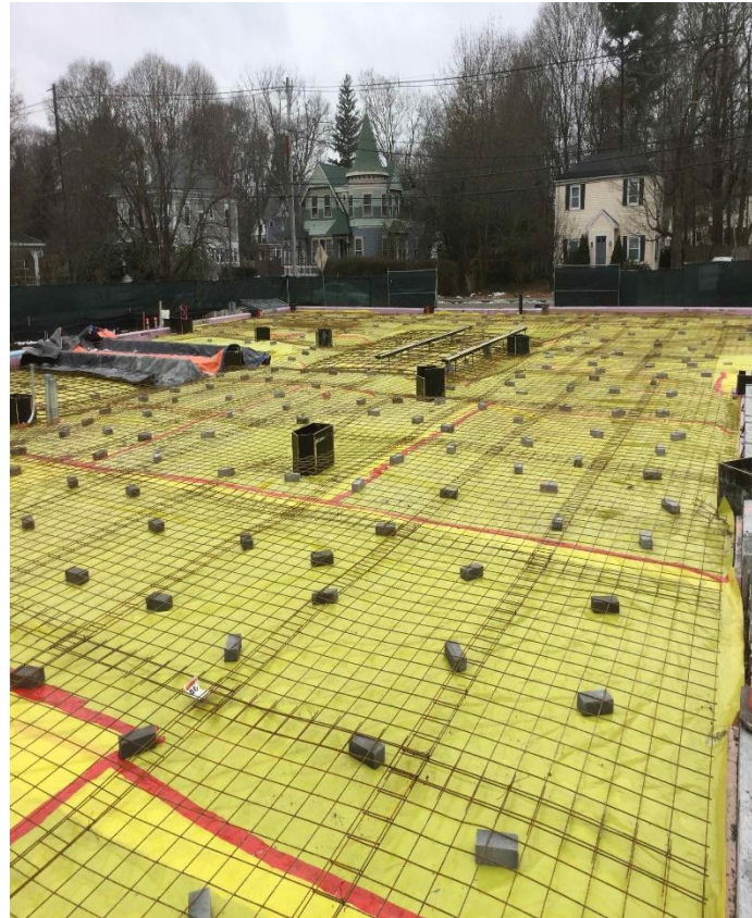
Slab Reinforcing
