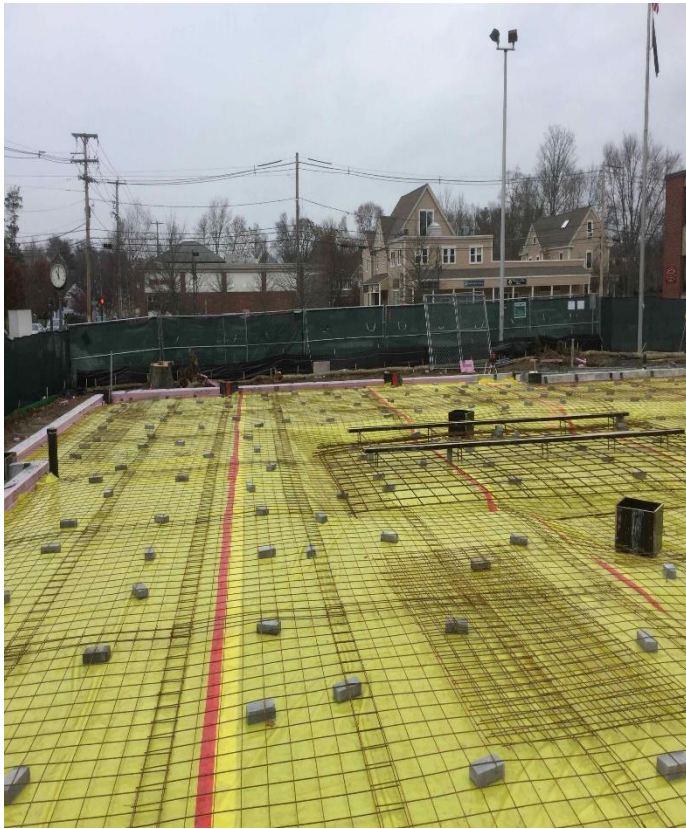
Slab Reinforcement
