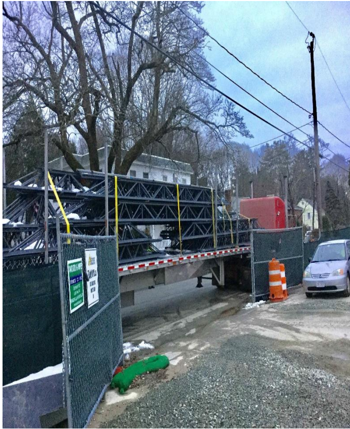
Steel Joist Delivery
