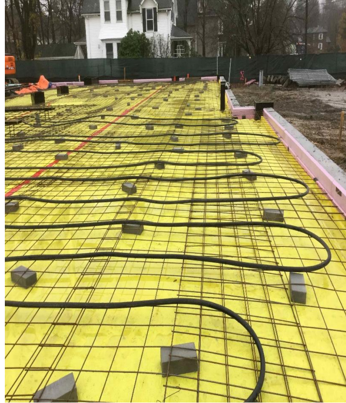
Ground Thaw Install
