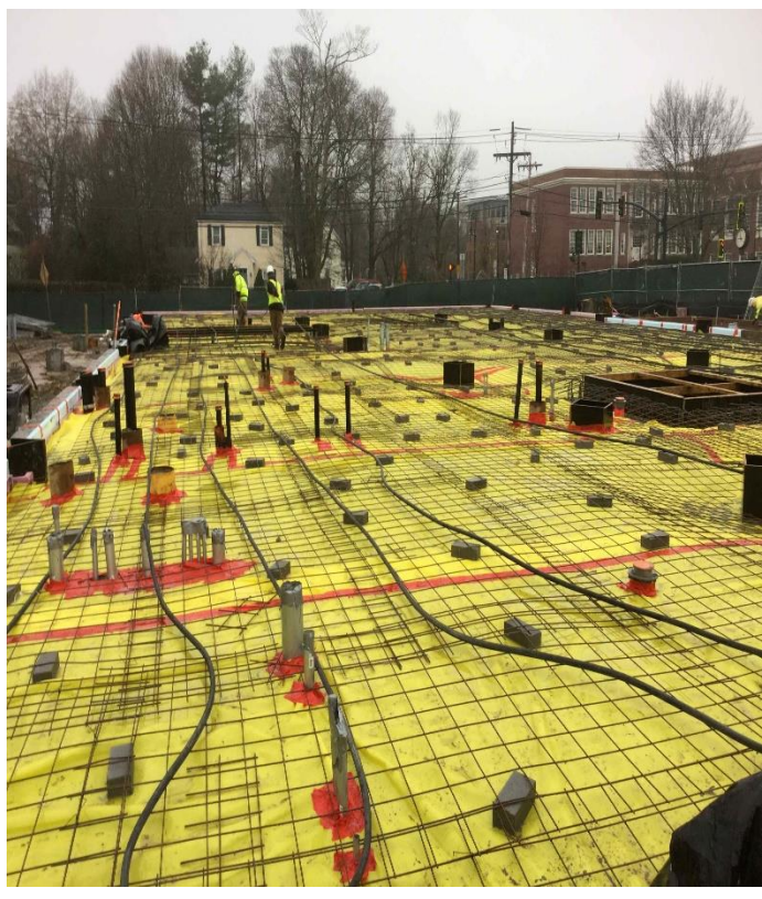
Ground Thaw Hosing Install
