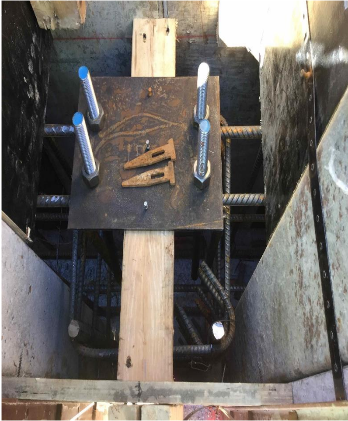
Rebar/Anchor Bolt Install
