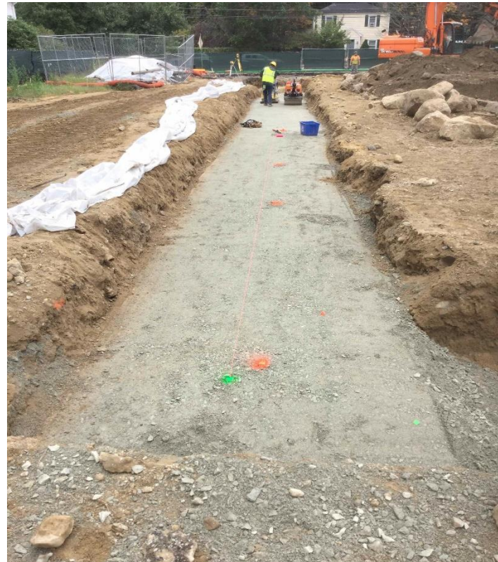
Structural Fill Subgrade
