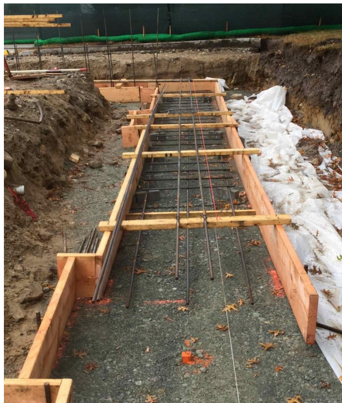
Footing Reinforcement 1 Line
