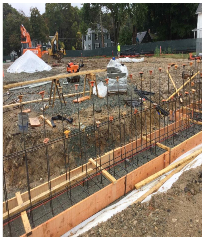
Footing Reinforcement A Line
