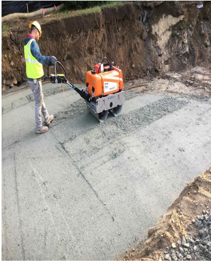
Structural Fill Compaction
