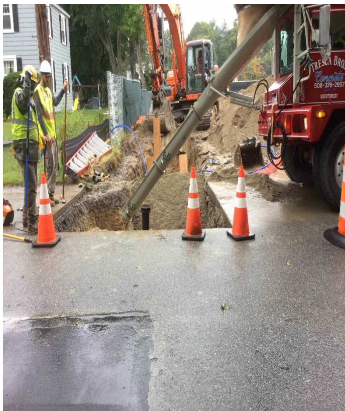
Backfill Street Trench
