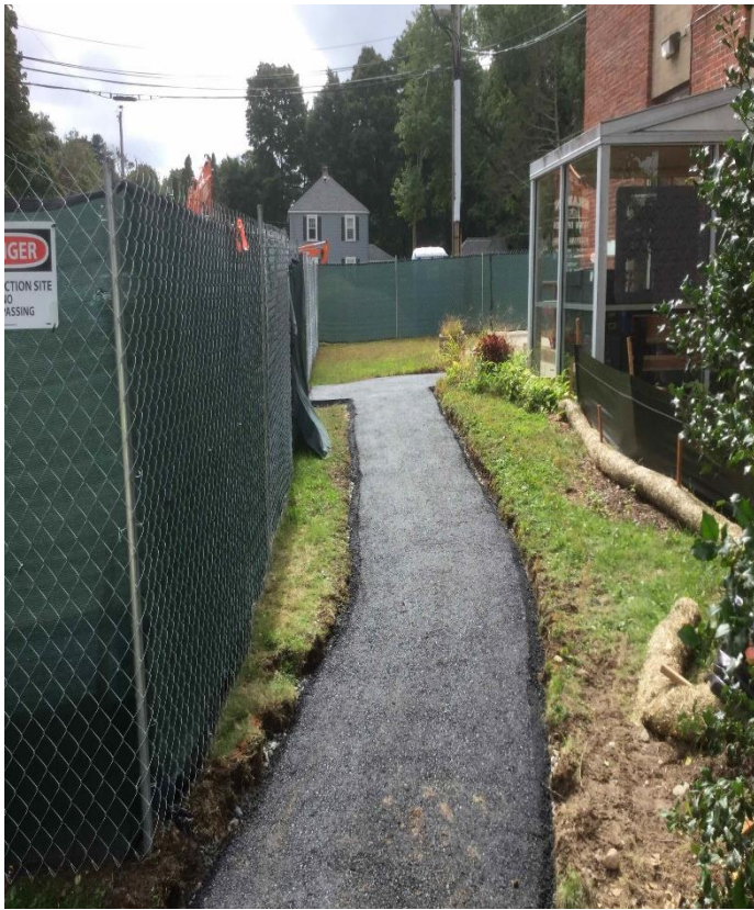
Temp. Asphalt Walkway
