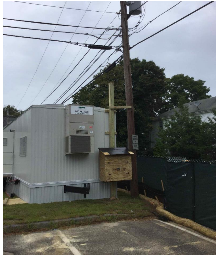
Temp. Electric Mast
