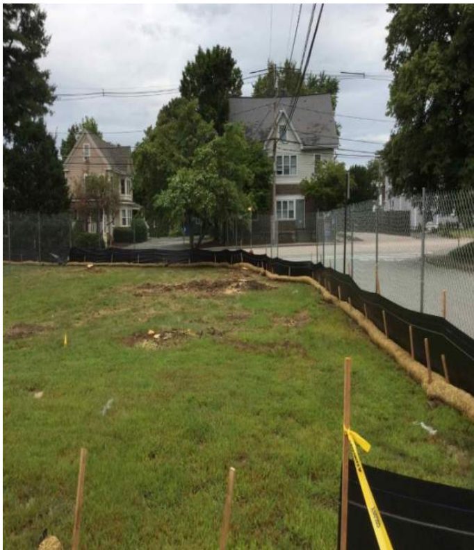
Fencing and Erosion Controls
