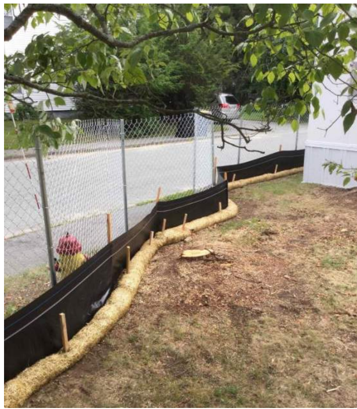
Fencing and Erosion Controls
