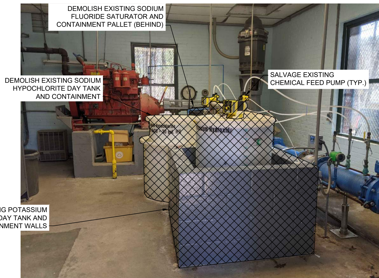
PICTURE 1 (P1) - WELL STATION 4 DEMOLITION
