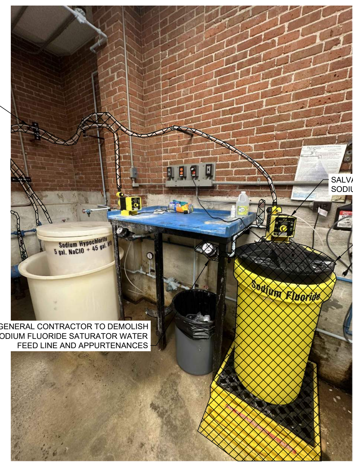
PICTURE 1 (P1) - WELL STATION 2 DEMOLITION SCALE: N.T.S.
