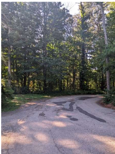
Photo 4: Overview of Well 4 Potential WTP location looking South
