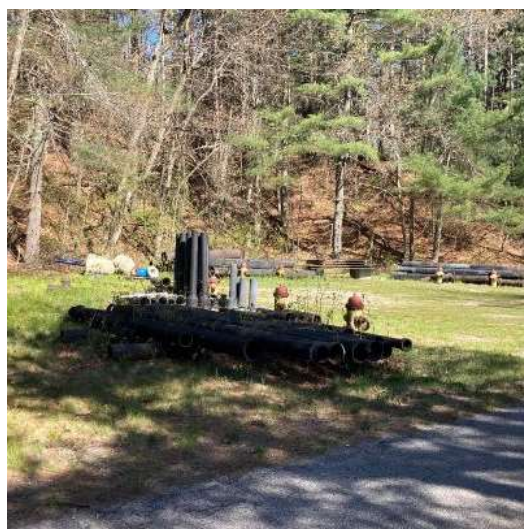
Photo 1: Overview of Well Station 2 Clearing Site
