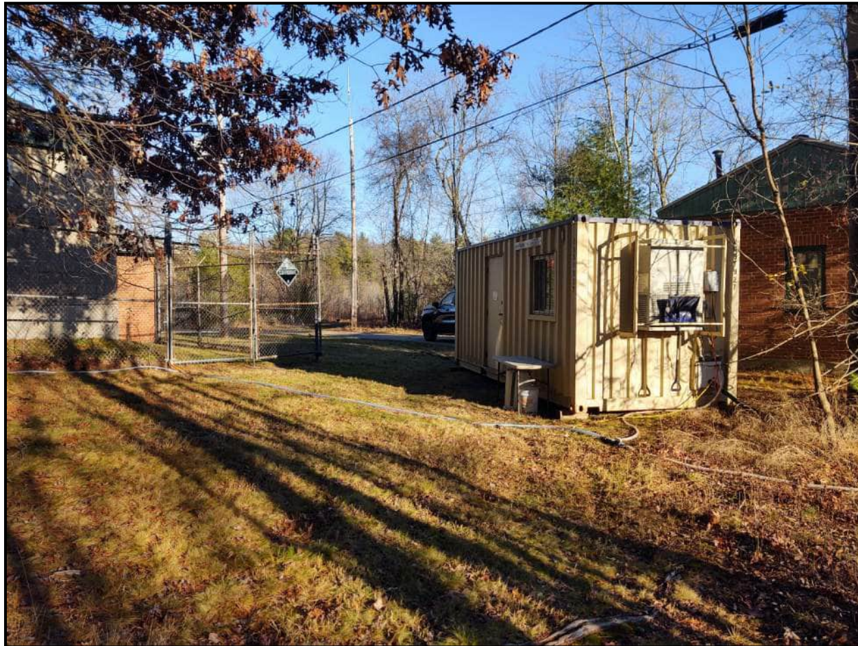
Figure 2.04: Ground Level Storage Container with Biological Pilot Equipment
