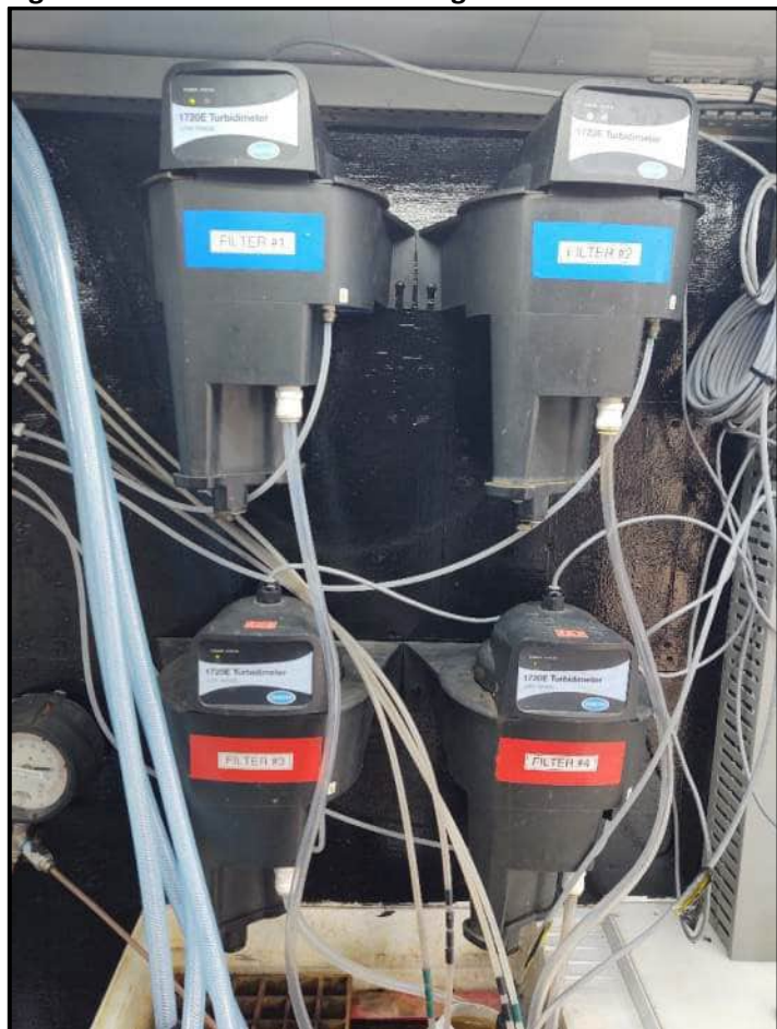
Figure 2.19: Hach 1720E Low Range Turbidimeters
