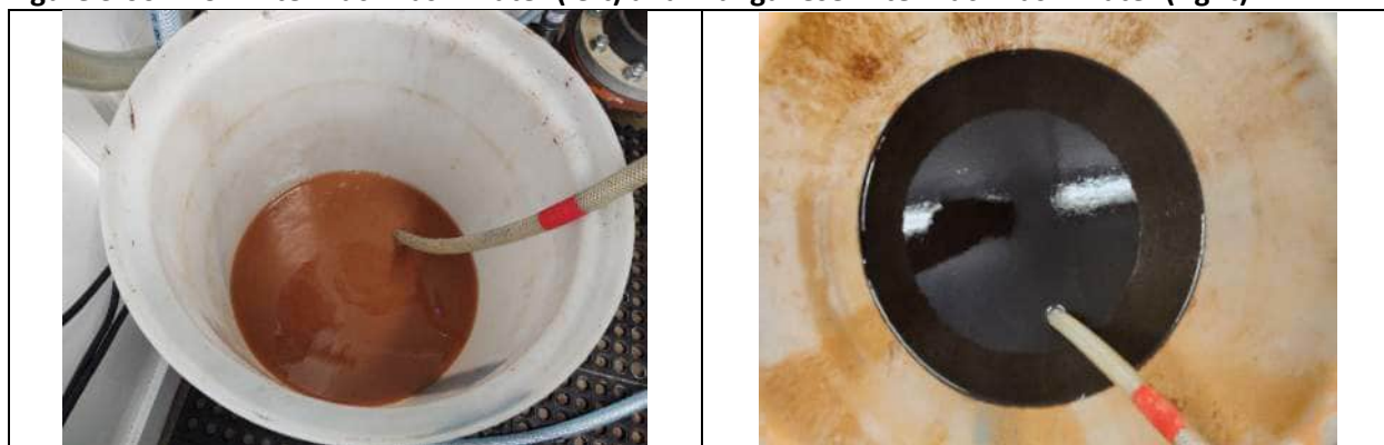
Figure 3.06: Iron Filter Backwash Water (left) and Manganese Filter Backwash Water (right)
