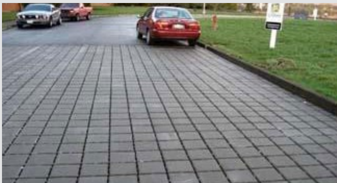
Example of permeable pavement that can treat and/or store rainwater where it falls. Source: https://www.epa.gov/green-infrastructure/what-green-infrastructure
