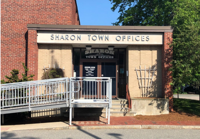
Existing Sharon Town Offices
