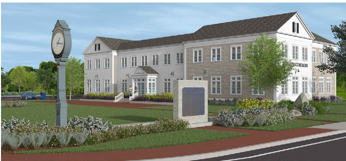
Figure 30: Sharon Town Hall Project
