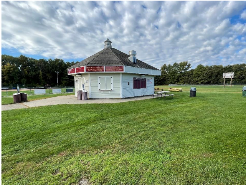
Deborah Sampson Field, Septic System and Snack Shack
