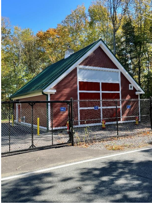
Emergency MWRA Pump Station
