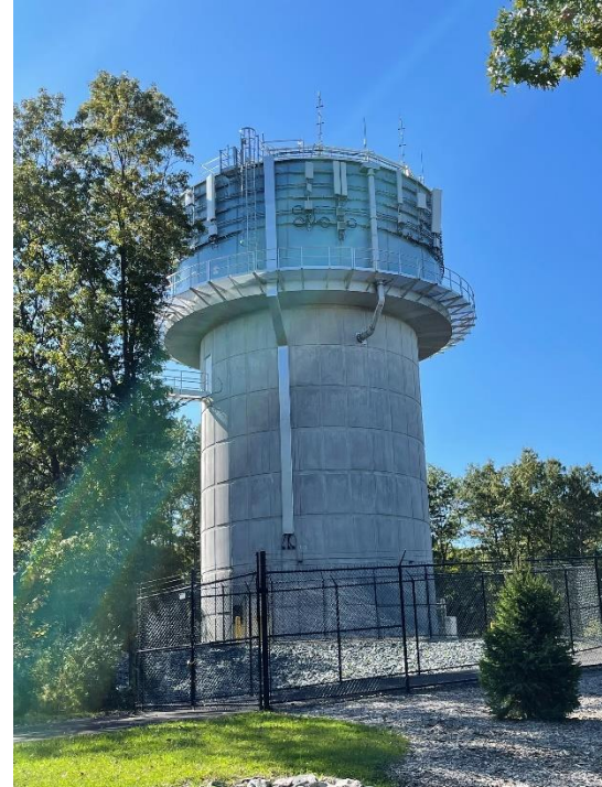
Massapoag Avenue Tank
