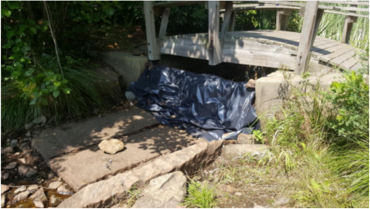
Figure 1. The non-permeable barrier in place at the lagoon spillway (08/05/18).
