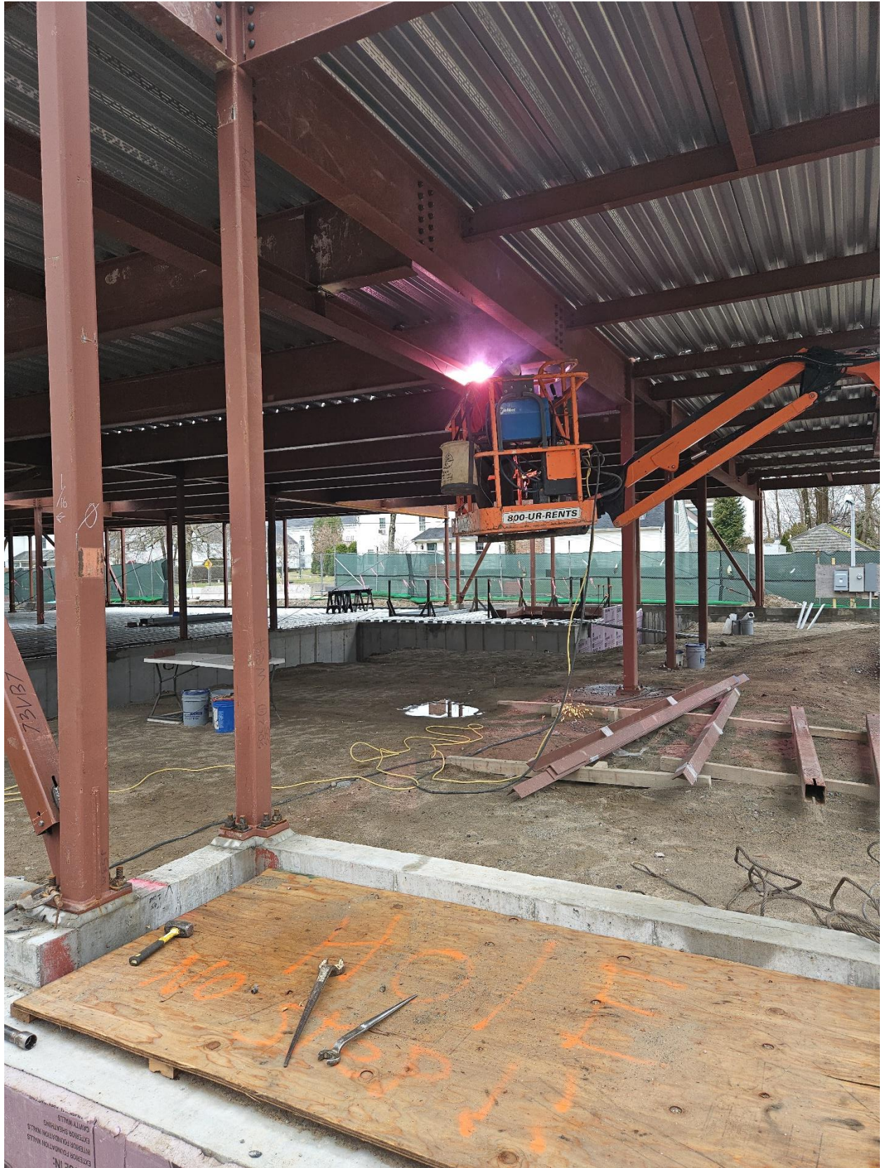
04.03.24 Welding Steel Connection
