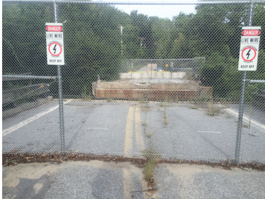
Photo 1 – Looking west from the east approach toward the west abutment.
