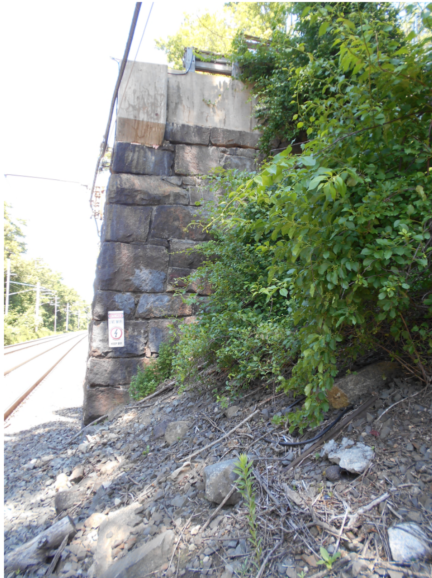
Photo 9 – Southeast retaining wall at the east abutment. Grades slope upwards to Maskwonicut Street. Thick vegetation is present.
