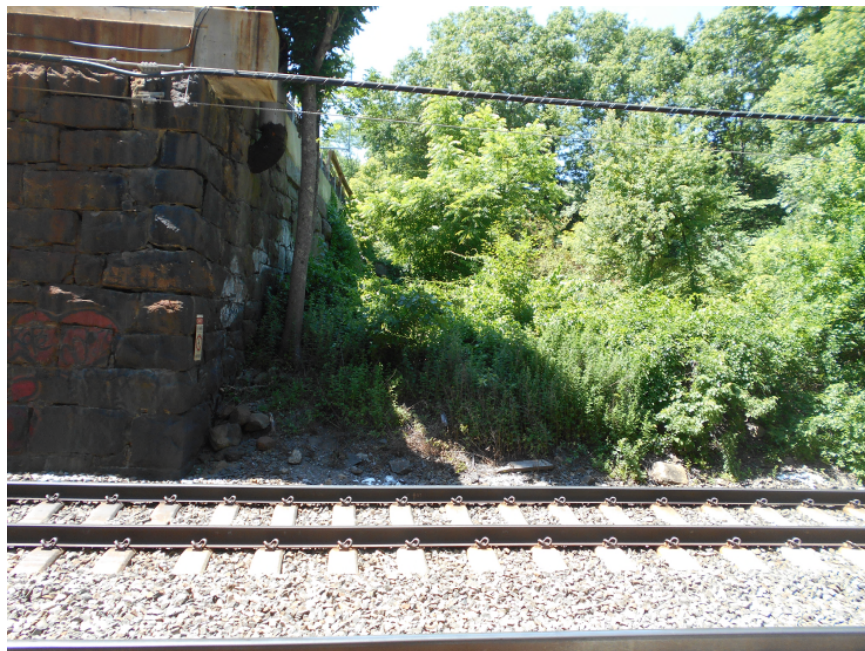
Photo 8 – Northwest retaining wall at the west abutment from the east side of the MBTA tracks. An earth berm is located between the tracks and Beaver Brook.
