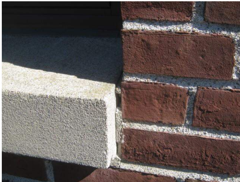
Spalled mortar joint
