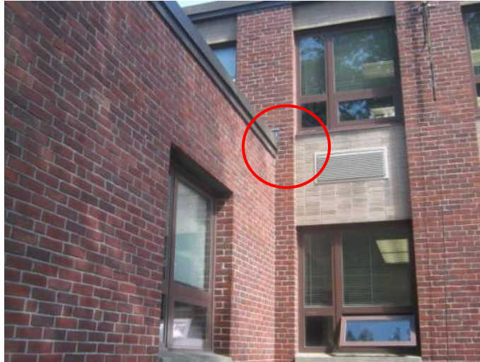
The south east corner where a diagonal crack developed in the brick wythe
