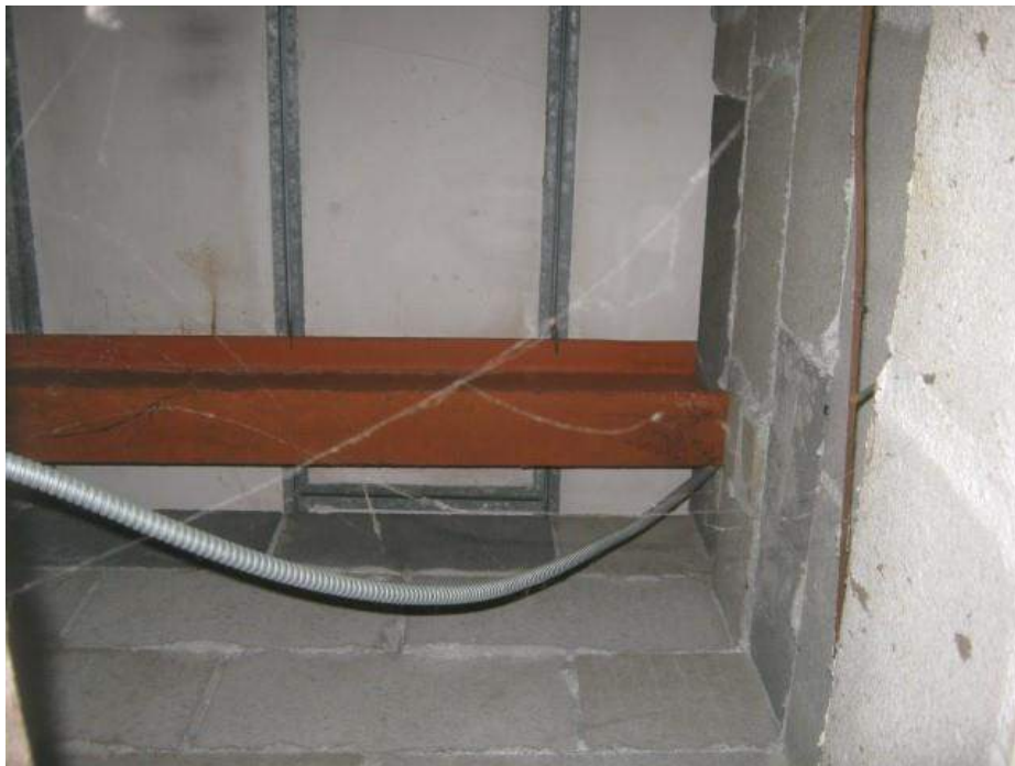
Gypsum prefabricated roof panels supported by steel beam
