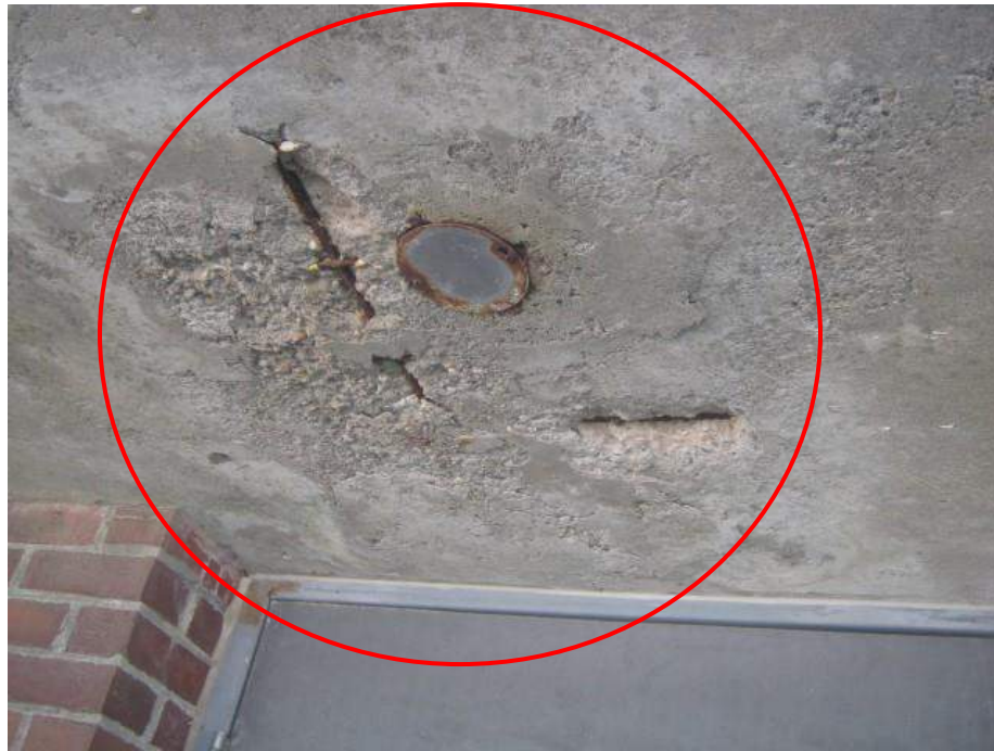
Exposed corroded rebar and spalled concrete surface
