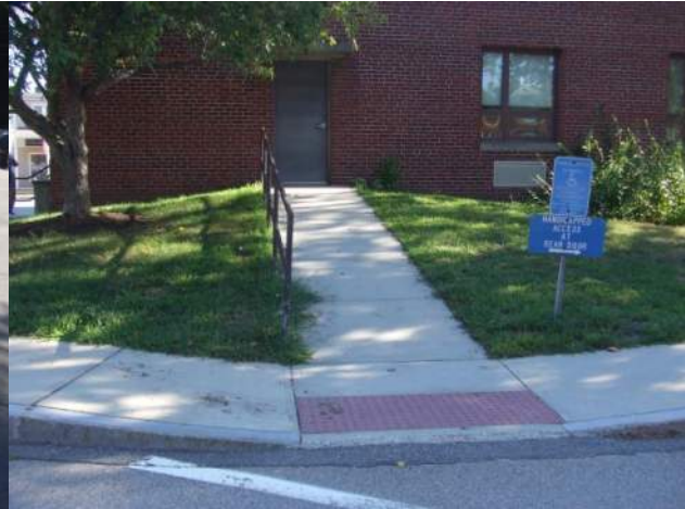
Ramp to building at 15.6% slope
