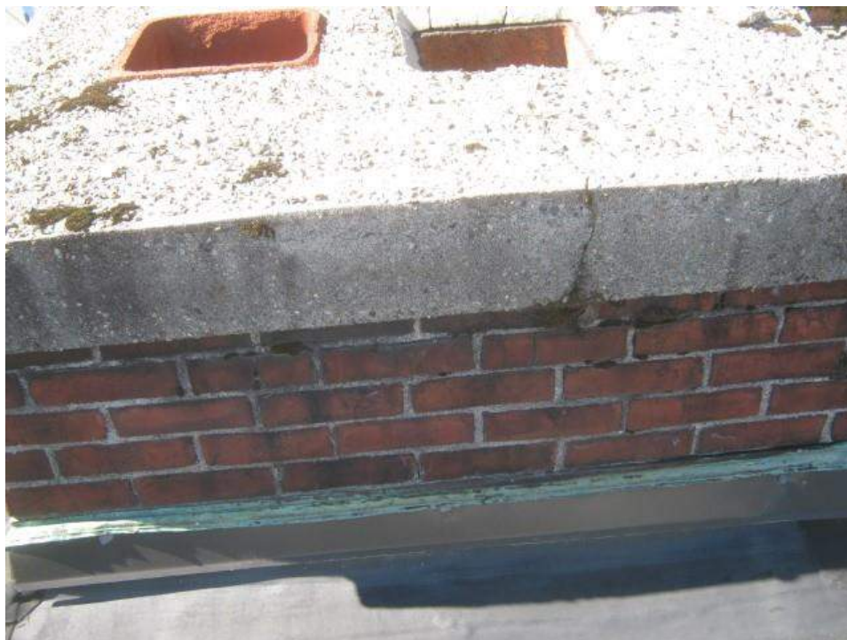
Vertical Cracks in the concrete cap on the north side of the chimney
