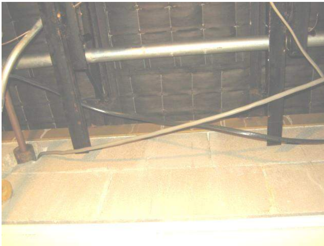
View of steel joists bearing on interior masonry bearing wall
