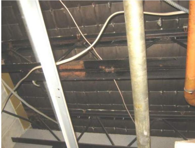
Floor Framing with Steel Joists and slab viewed from the underside
