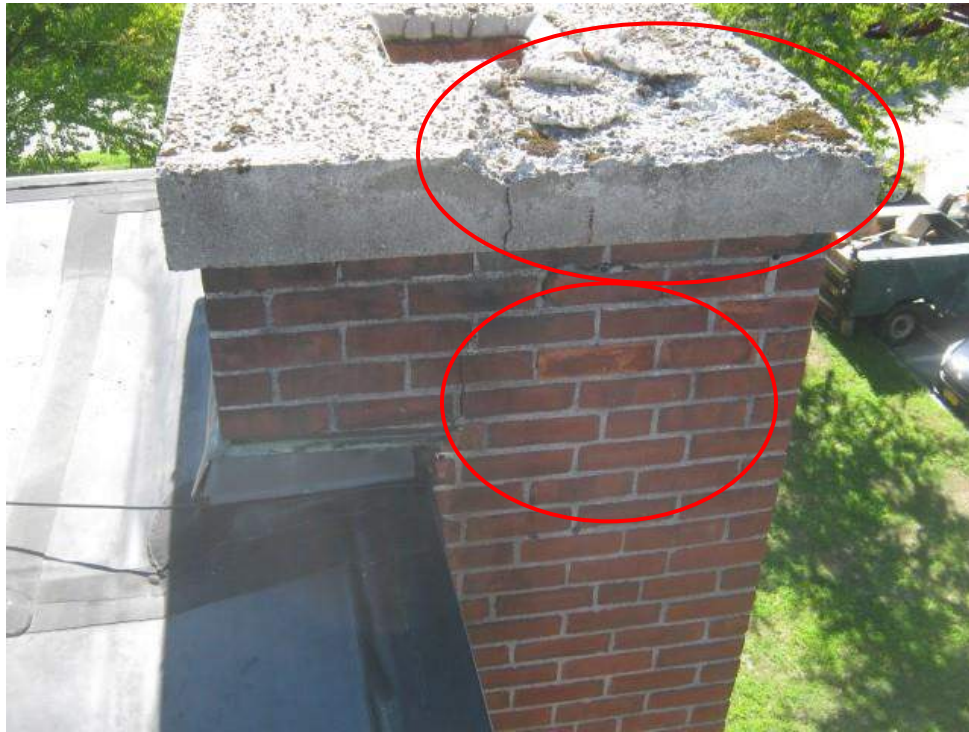
Cracked and Spalled concrete cap and brick
