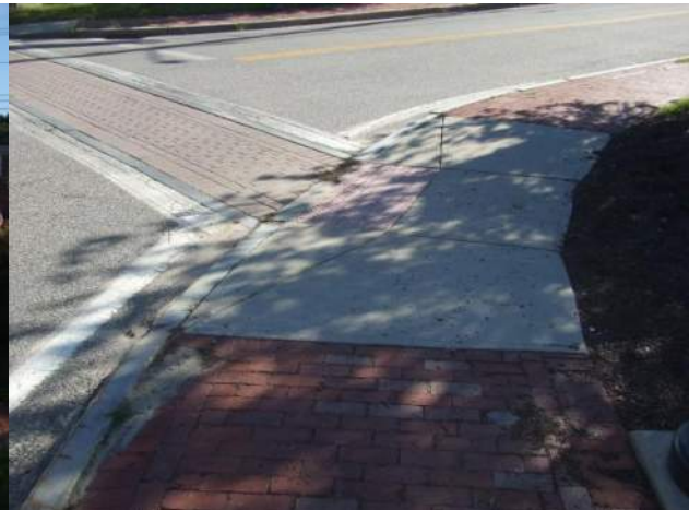
Curb cut at South Main and E. Chestnut
